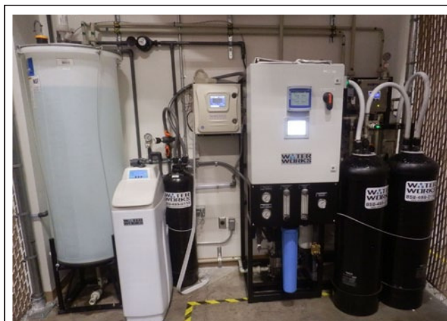
Figure 6. System I2 with single HRC UV reactor.
